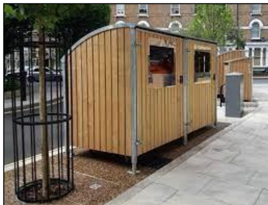
Example of practical and more attractive bin storage
